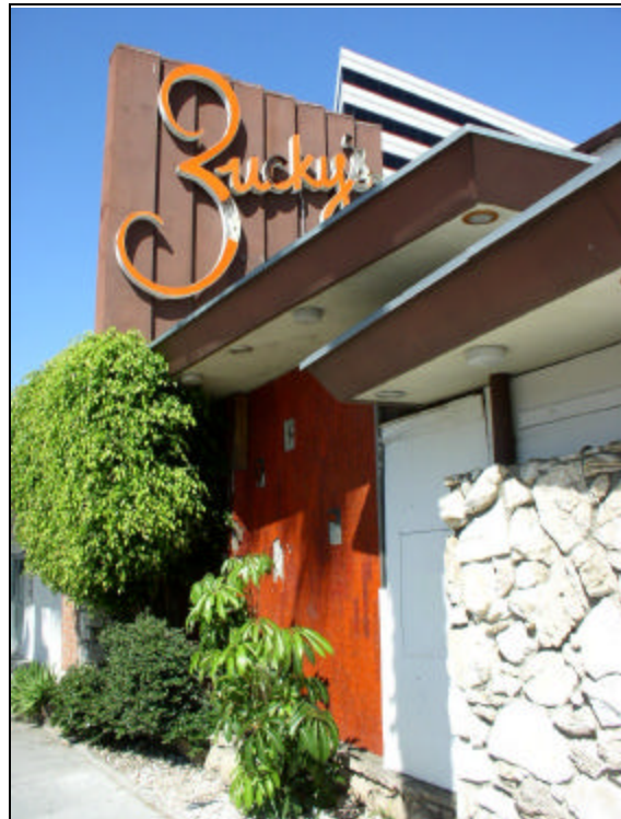
East elevation, looking northwest.
