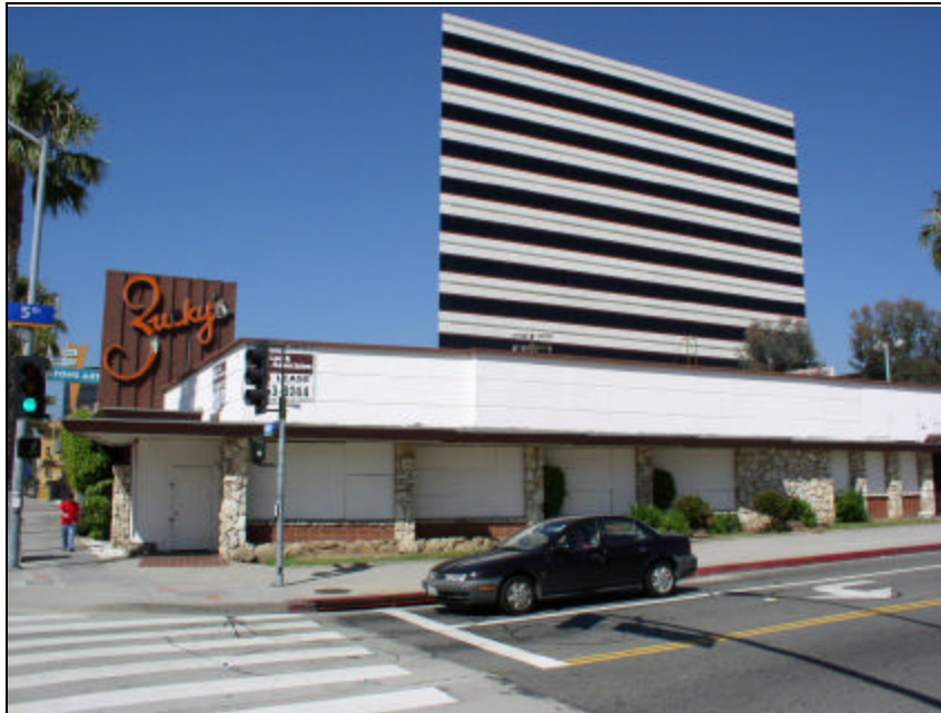
Primary (east) elevation, looking northwest.
