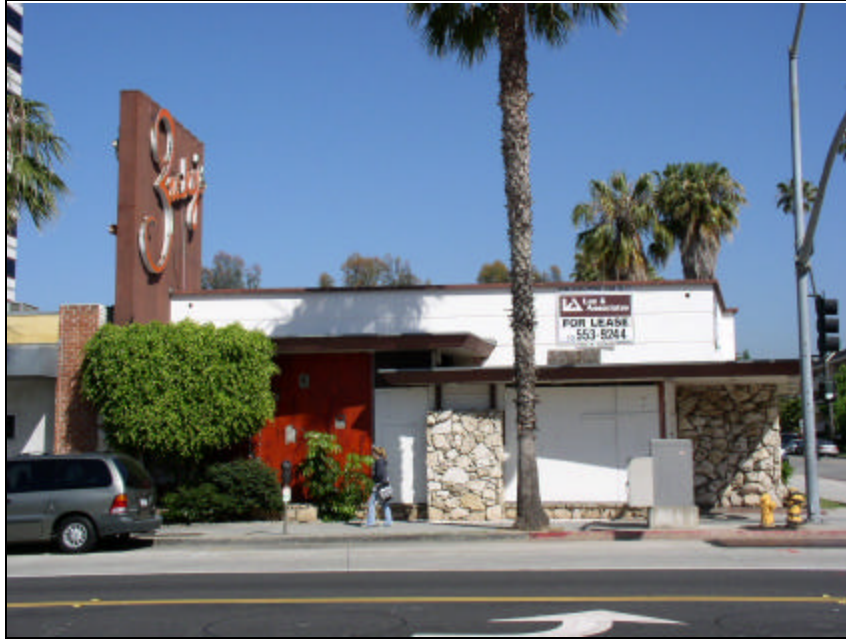
Primary (south) elevation, looking north.
